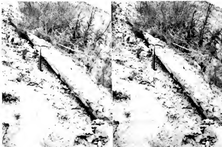
Photo 6. A stereoscopic photo of the break on bedding planes in the Sunshine Ranch Member of the Saugus Formation in a freeway cut just east of Lower Van Norman Reservoir (57).
